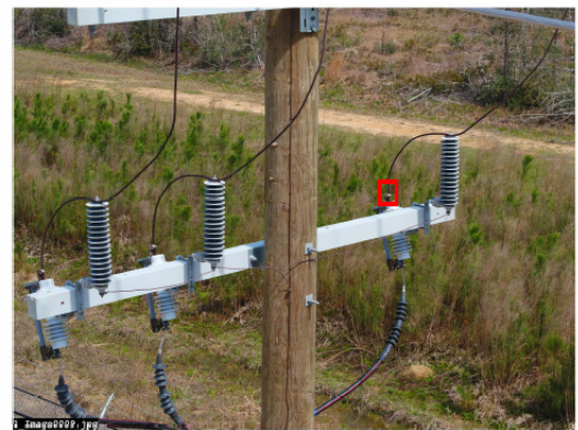
Tower 11: Loose conductor strands
