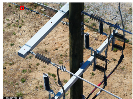
Tower 17: Loose cotter key
